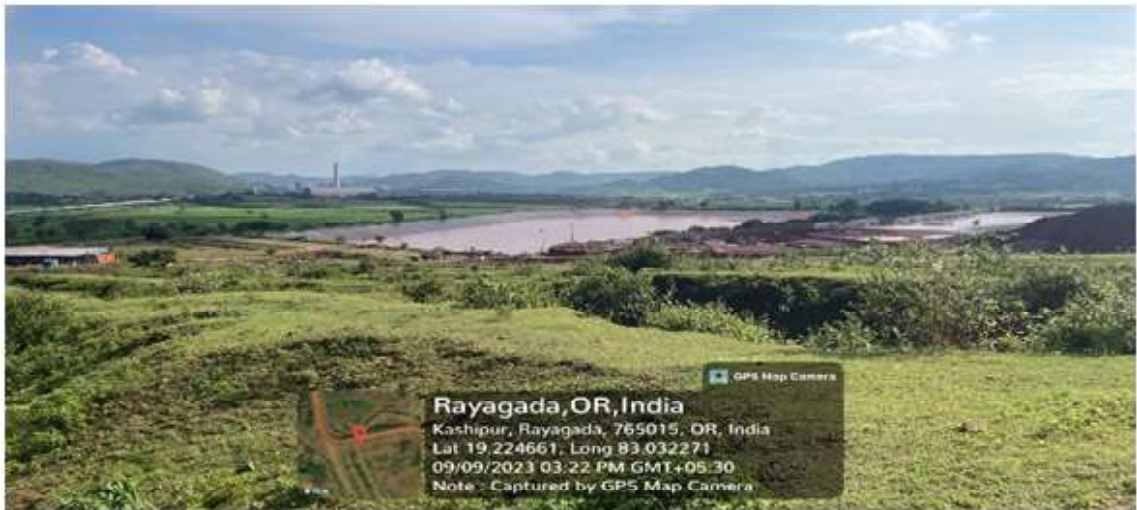
Figure 14: Red Mud dewatering Pond
